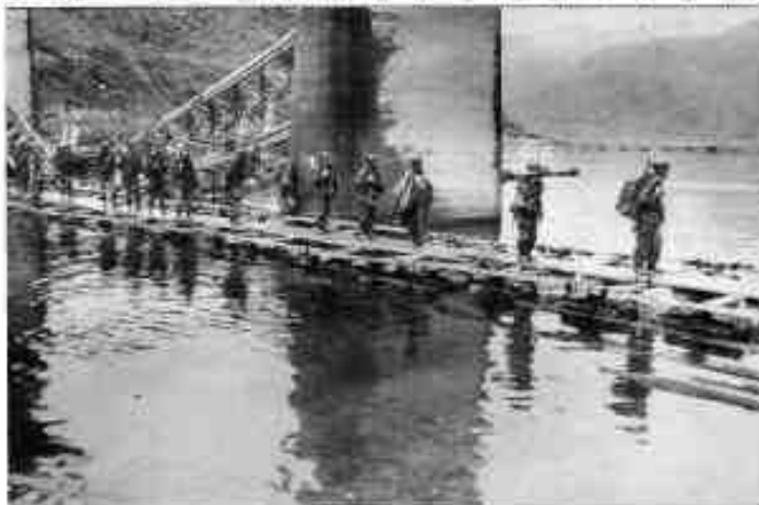
ENGINEERS CROSS THE HANRIVER ON A TRESTLE BUILT IN SHORT ORDER OF EMPTY 55 GALLON DRUMS AND PLANKS. JUNE 1950 Photo by Norm Strickbine
