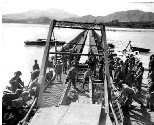
Engineers assemble a ponton bridge near Waegwan Korea September 22 1950
